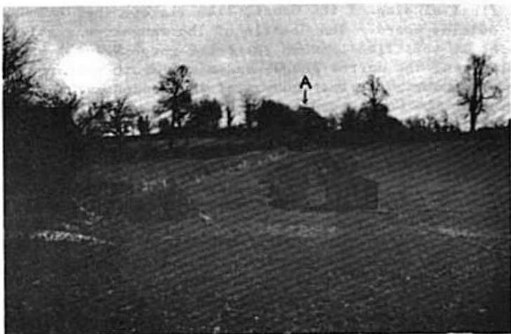
1. ILMINSTER INCLINE. Incline, now straddled by low hedge, continued behind hedge, left foreground, into lower pound of canal. Cutting at top of incline leading to tunnel is just visible (A).
